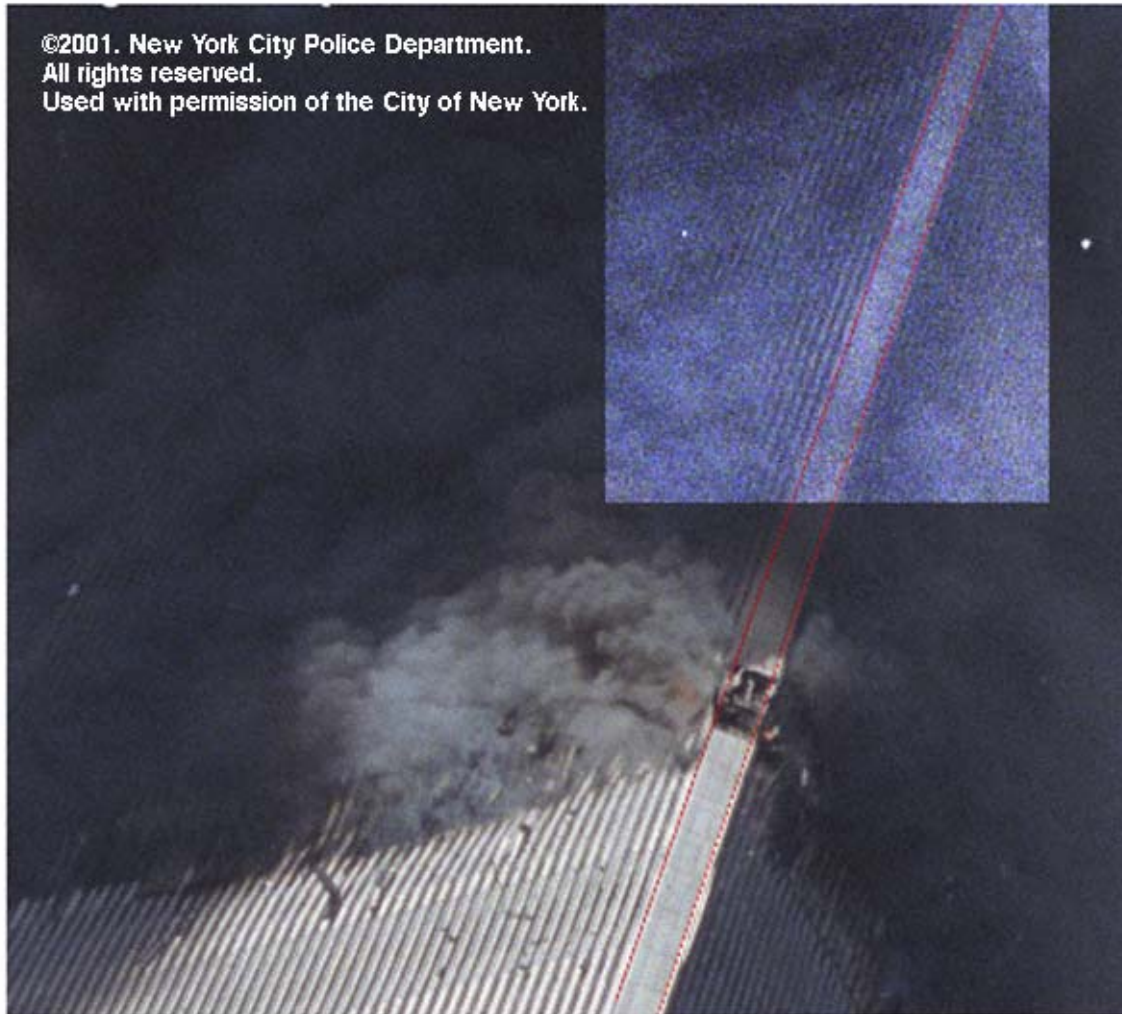
Figure 6–21. Northeast corner of WTC 2, several seconds before collapse. The corner shows no distortion of the type in the previous figure, implying that the distortion accompanied the collapse and did not precede it. The region in the upper right is enhanced for visibility.
