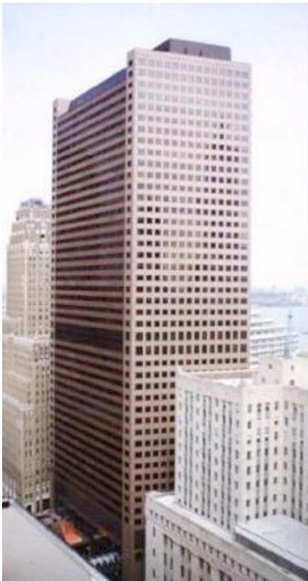
WTC 7: 47 - Story, steel-frame building..
